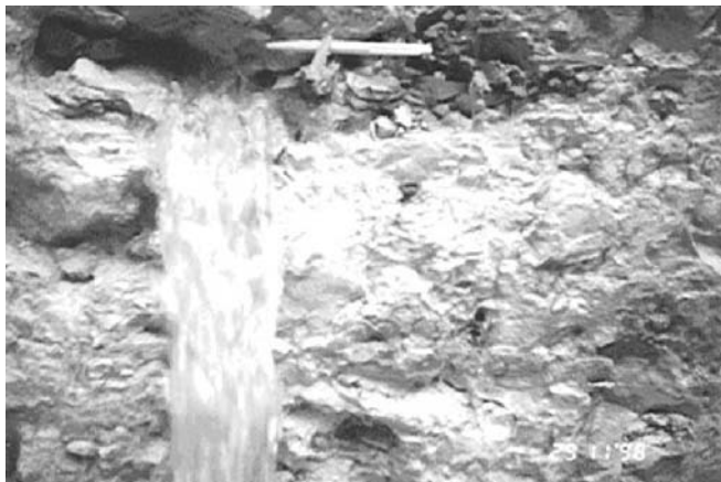
Fig. 2 General view of the trial pit with submersible pump
