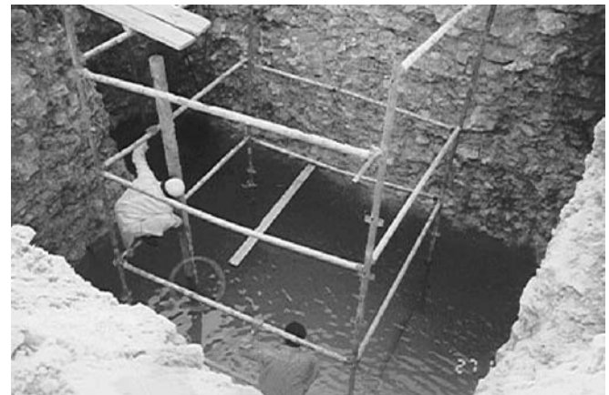
Fig. 7 Measurement of water levels, in the nonsteady-state condition
