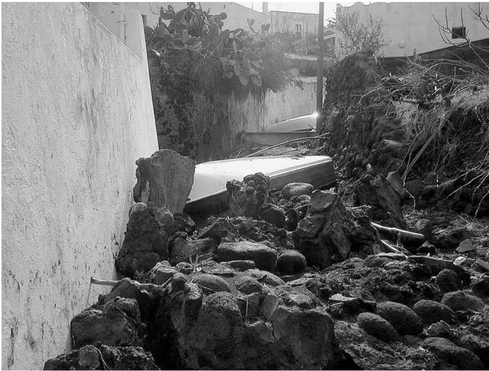
Fig. 9 Photo showing small boats, broken walls and debris carried by the tsunami waves and channelled along one of the narrow streets of Ficogrande. The picture was taken during the second of the three surveys (21–23 January 2003)
