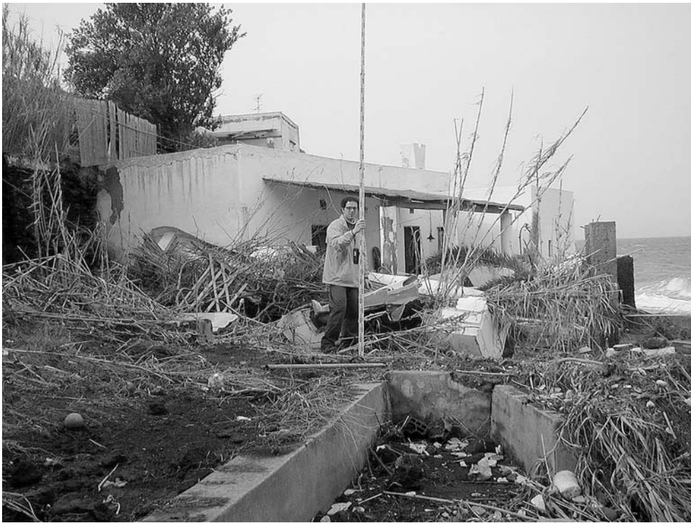
Fig. 8 Flattened vegetation, small boats carried inland, and small walls toppled down as observed in one of the houses at the northwestern end of Piscità. The picture was taken during the first of three surveys (11–13 January 2003)
