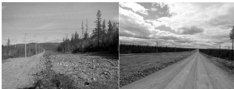
Fig. 6. ESPO sections with an organized technological highway along the pipeline in the conditions of continuous distribution of permafrost. Photo by S.I. Serikov.
