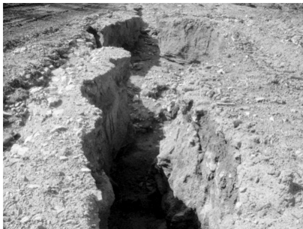
Fig. 1. Frost fissure along the ESPO pipeline. Photo by L.A. Gagarin.
