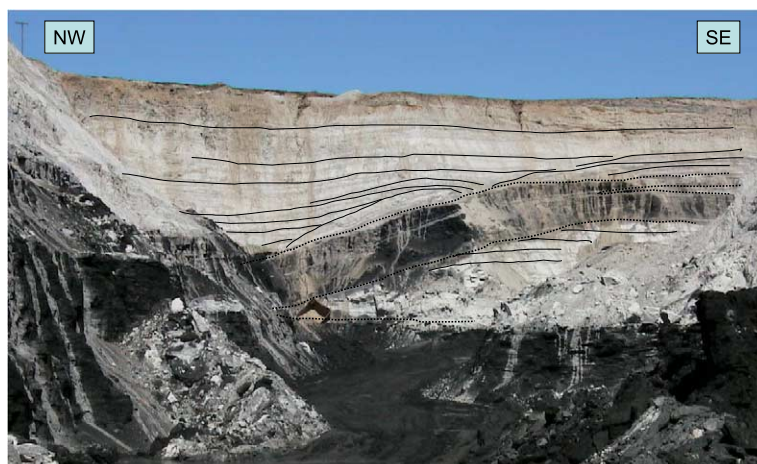
Fig. 8. SE–NW cross section along the northeastern slope of the Baganuur open pit. The photograph shows the contacts between the lower coal seam and roof and floor rocks as well as seam split (dotted line). Bedding planes and bounding surfaces within the interseam sediments are highlighted by heavy lines.
