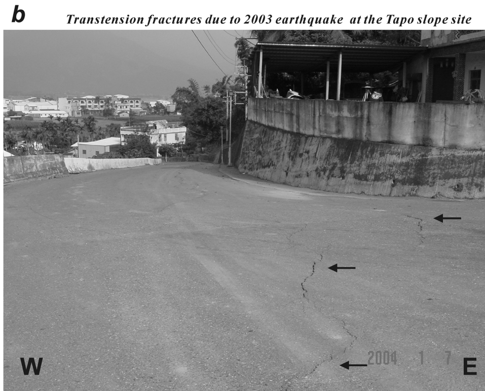
Figure 4. Photographs of the surface ruptures of concrete pavement along the roadside caused by the 2003 Chengkung earthquake at the Tapo slope site. (a) Pop-up-type or reverse fault-type fractures that indicate compression or shortening. (b) Open en échelon fissures (indicated by arrows) that show transension from near the top of the geomorphic scarp.
