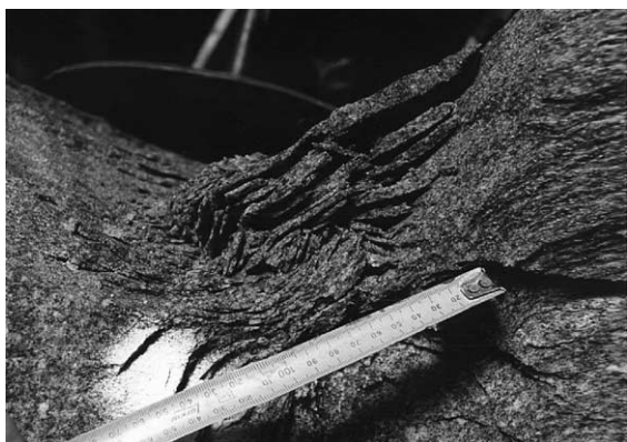
Fig. 6. Photograph of lower notch, exposed by excavating a trench in the floor.
