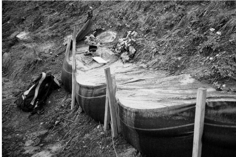
Fig. 6. Eroded sediment accumulated upslope of a silt fence installed following the Bitterroot Fire in 2000 in Bitterroot National Forest, Montana, USA (photo courtesy of Kevin Spiegel).
