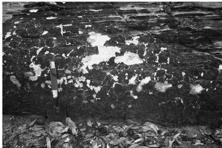
Fig. 1. Weathering of Hawkesbury Sandstone bedrock, Nattai National Park, New South Wales, Australia, caused by wildfire in December 2001. Lighter-toned patches indicate where lensoid-shaped flakes have been removed. The contrast in tone between these patches and the remaining dark rock surfaces suggests that the flakes were removed after the fire. Note hand trowel for scale.
