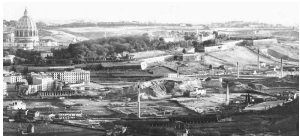
Fig. 2 View of the “Valle dell’Inferno” valley in the 1910s from Monte Mario hill (see Fig. 1): to be noticed are the chimneys of the clay kilns and the scarps of the quarries of “Marne Vaticane” stiff clays
