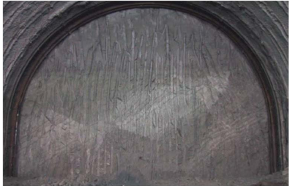
Fig. 8 Excavation front of the “Passante a NW di Monte Mario” tunnel: note the transgression of the Monte Mario unit over the “Marne Vaticane” unit and the tectonisation of the “Marne Vaticane” unit ( red lines )
