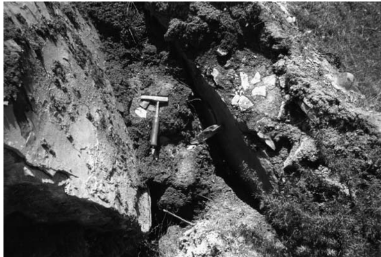
Figure 4. Example of fractured sandstones constituting the slopes of the Valderchia landslide.
