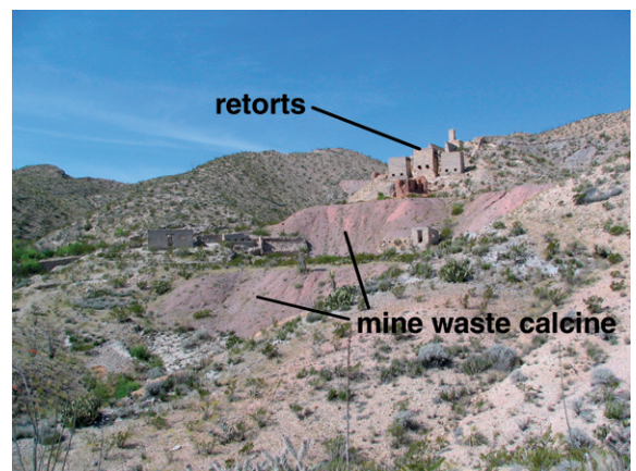
Fig. 2. View of the inactive Mariscal Hg mine located in Big Bend National Park. This was the smallest mine studied and it produced about 50 t of Hg during mining from 1900 to 1943. There are presently about 3 \times 10^4 \text{ m}^3 of mine waste calcine at the Mariscal mine.
