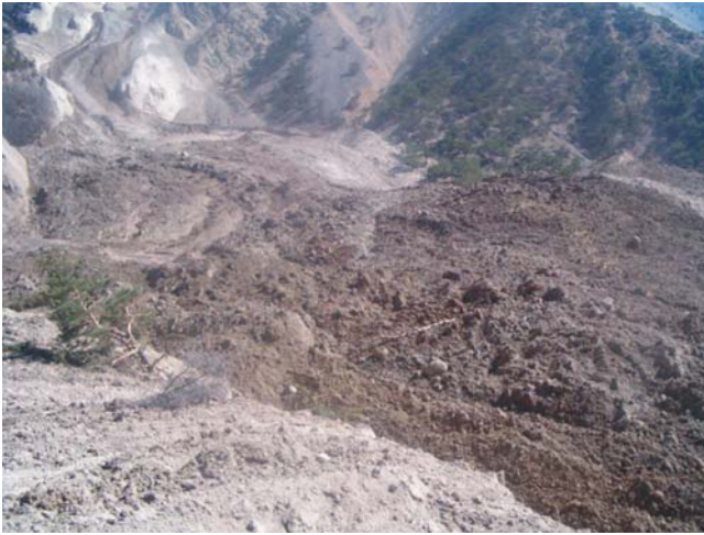
Fig. 5 Settlement area covered by debris material
