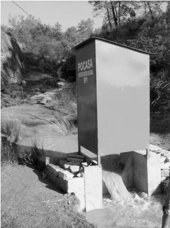
Fig. 2 Location of control station no. 5
