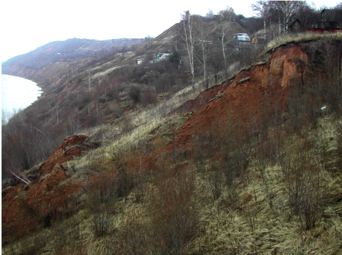
Figure 6. Landslide that collapsed from the high shore of the Oka River in November 2004.
