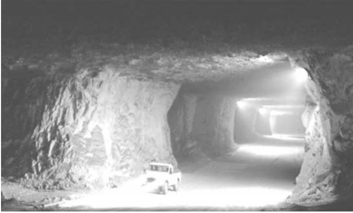
Fig. 3. Typical view of Middleton Mine
