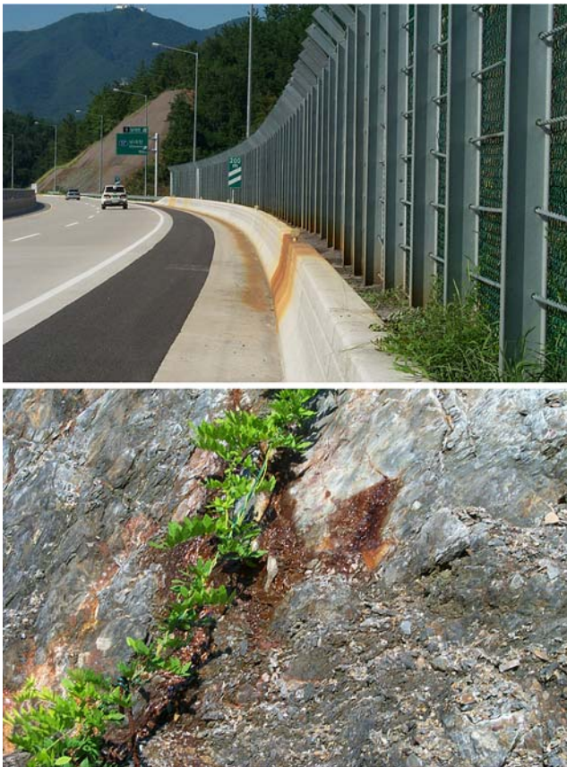
Fig. 2 Oxidation marks at the road cut slope in the vicinity of Mujoo area
