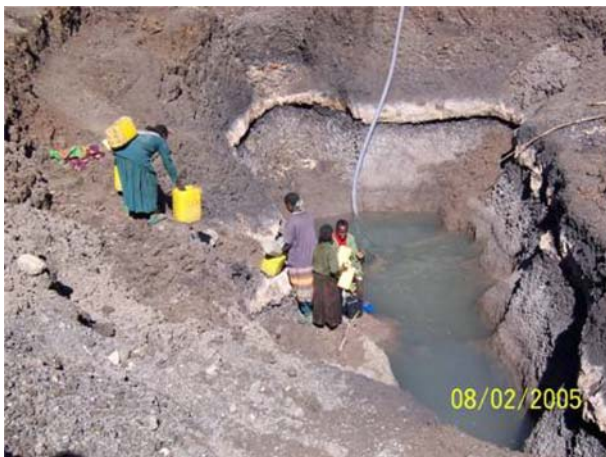
Fig. 6 Dug well at the center of dry lake basin. The water level is at the depth of 6 m
