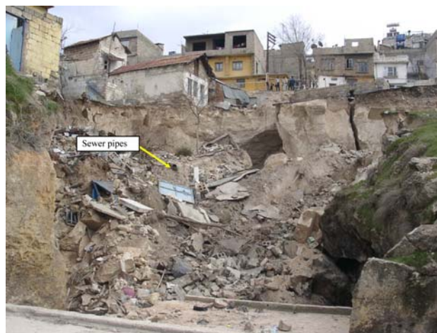
Fig. 4 General appearance of the collapsed cave near Karakabir
