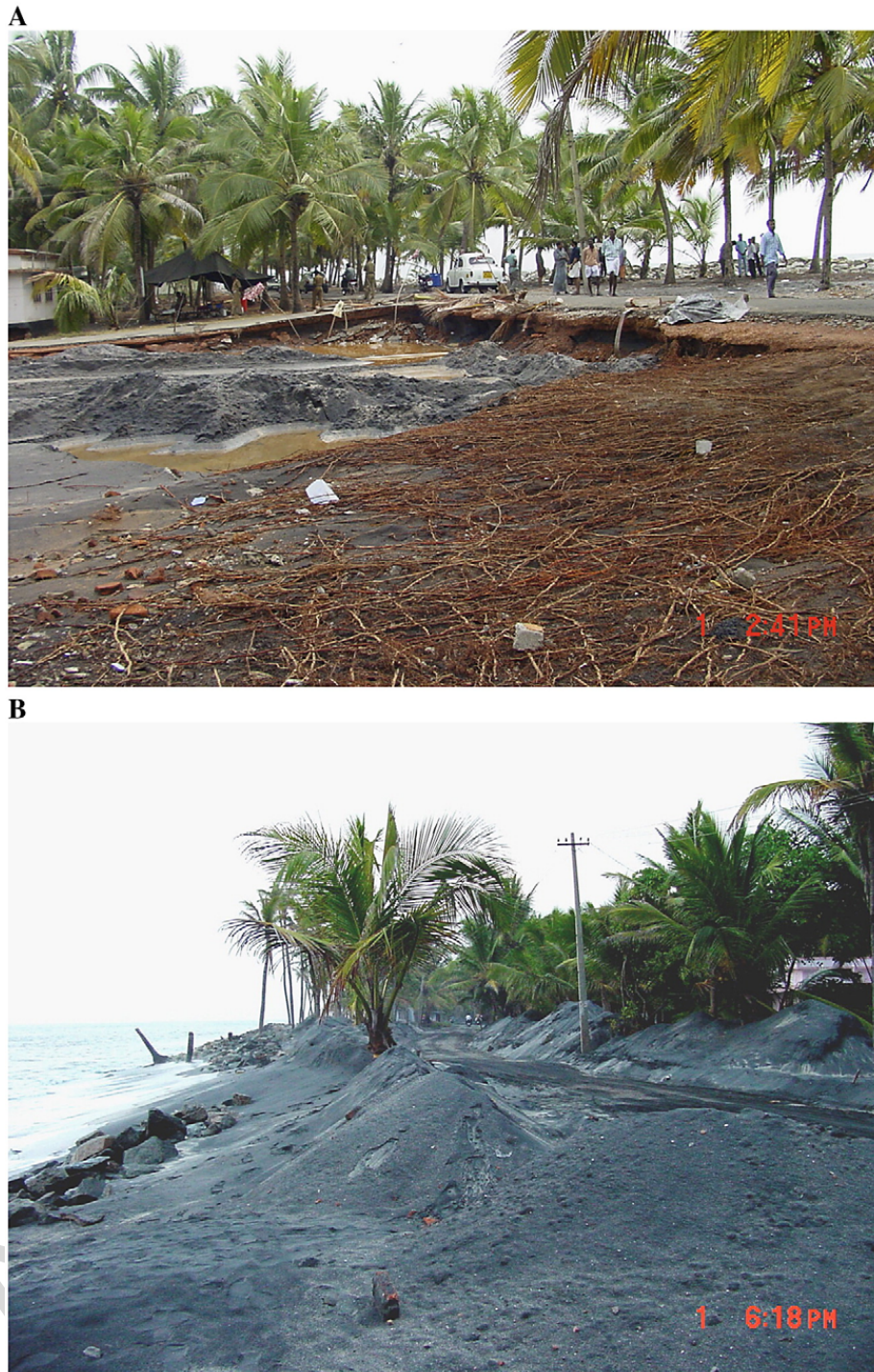
Fig. 5. Post-tsunami geomorphic features along the southwest coast of India. (A) Deep trench cut by the tsunami. Partially filled portion with coir and lateritic soil is seen. (B) Shore face altered by the tsunami and huge dump of black sands on the coastal road. (C) Inundation pathway of tsunami, transported seawall boulders obstructed by the coconut grove and thick black sand concentrates are seen. (D) Dump of black sands in the porticos of coastal homes. (E) Picture shows shore erosion on the northern side of Kayamkulam estuary, disfigured back-berm after the tsunami hit the coast. The displaced boulders from the sea wall are visible in the foreground.
