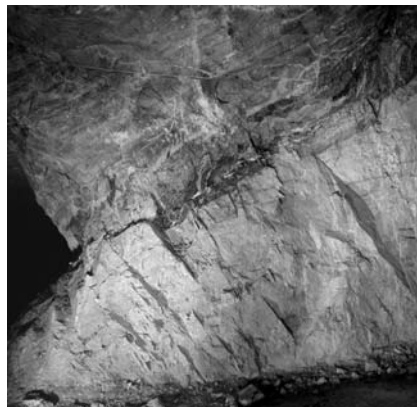
Fig. 19. Detail of the sliding plane of the serpentine filling in pillar GH89
