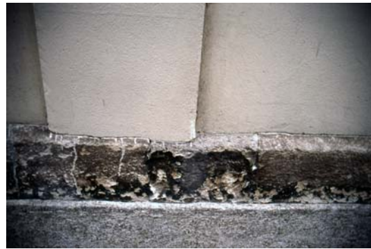
Fig. 2 S. Jorge church, La Coruña. Sampling area: granitic plinth at the base of the S-SW wall
