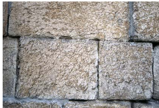
Fig. 4 S. Jorge church, La Coruña; weathered granitic stone surface showing exfoliation and scaling
