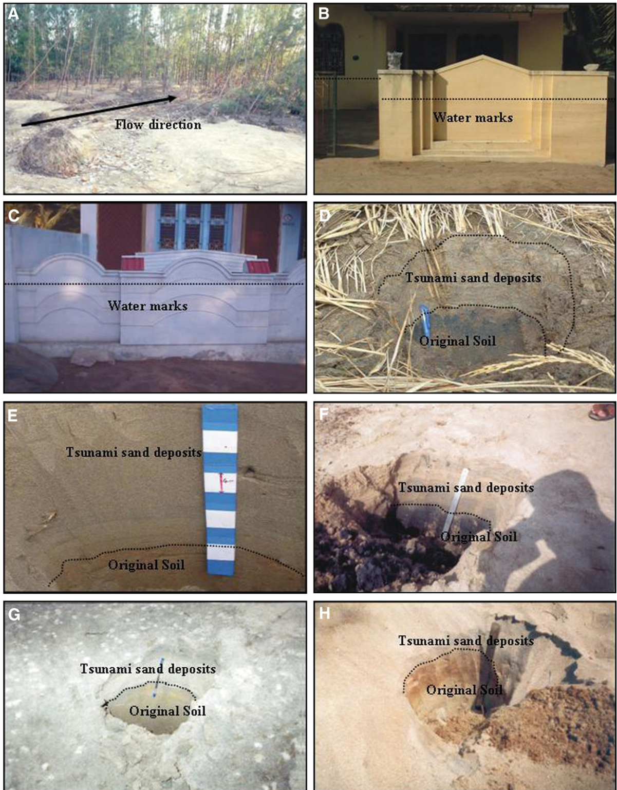
Fig. 2. The direction of water flow is marked with an arrow (A) and the water level can be observed on the white wall (B). Water level and considerable erosion is also noted in front of the concrete foundations (C). The tsunami deposits were generally identified as grey sands that overlies the soils of the coastal plain (D–H).
