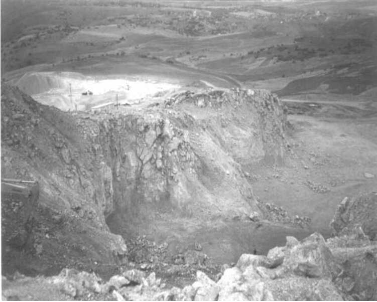
Fig. 5. Blasting area left in place
