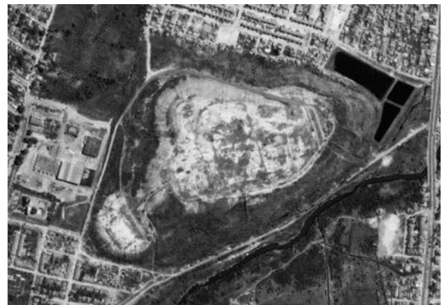
Fig. 15 Current conditions (vertical view) of the Jangurussu uncontrolled sanitary landfill. Control measures (surface drainage and covering system) implanted after 2004 are visible
