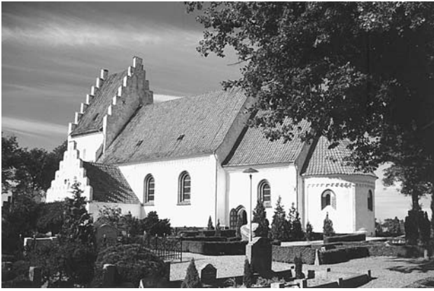
Fig. 1 View of Brarup Church from the southeast. The nave, chancel and apses are build of red brick masonry around 1300. The church is situated at the island Falster close to the Baltic Sea
