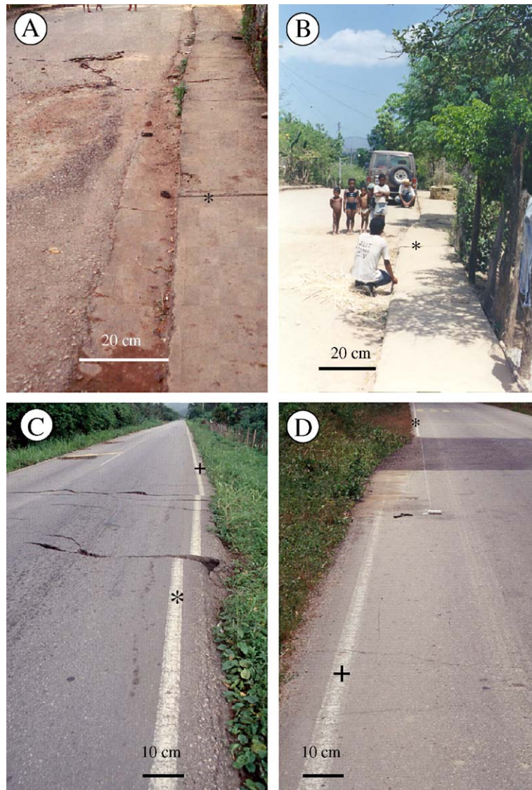
Fig. 10. Comparison of dextral slip between in the first week after the Cariaco 1997 earthquake and 5 months later (December 97), at Terranova (A and B) and at national road 10 west of Casanay (C and D). Total slip at both sites (B and D) roughly doubles the initial coseismic slip (A and C);
