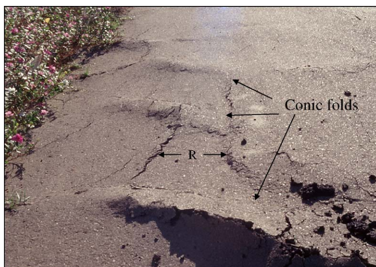
Fig. 7. Ground view of en echelon conic folds at restraining stepovers between adjacent R shears in lateral yard of Las Manos hardware store, next to flower buckets in Fig. 3.
